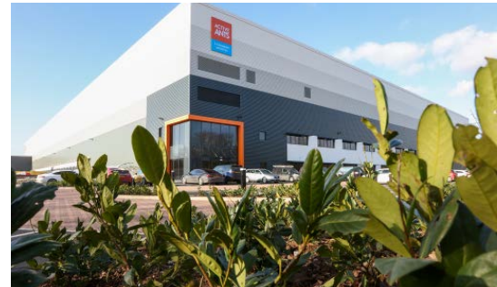
03 BRACKMILLS GATEWAY NORTHAMPTON, A45
